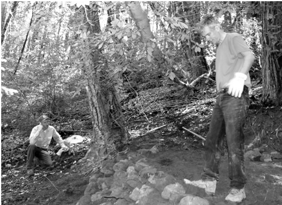
Josh Moore works with MROSD staff to construct a retaining wall on the Crossover Trail in El Corte de Madera Open Space during a trailbuilding project in 2005
