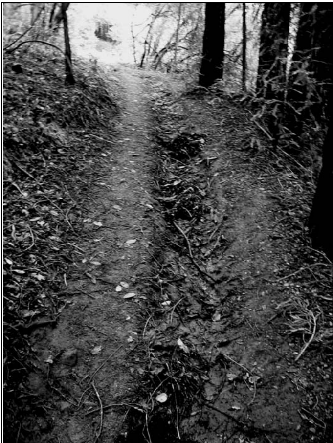
Equestrian trail use causes "troughing", an erosion pattern with a flat bottom, typically one foot wide, up to a foot deep.
